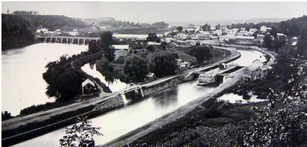
Historic photograph of the upper aqueduct carrying the Erie Canal across the Mohawk River near Schenectady.
